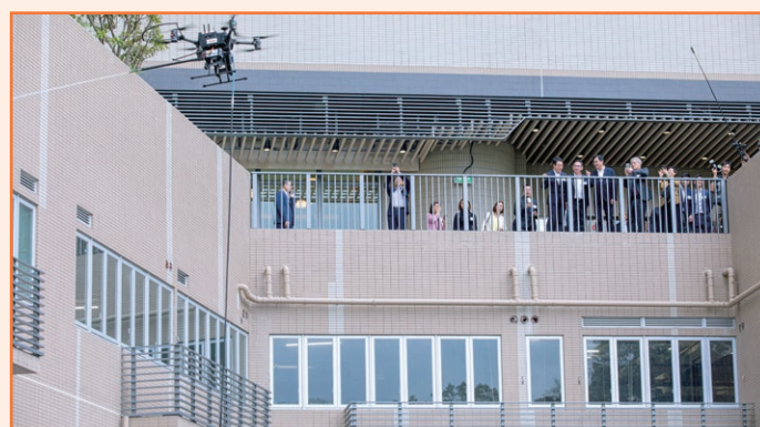
房協引入無人機技術清洗大廈外牆。無人機可高效且安全地到達難以觸及的外牆位置，協助樓宇保養工作。 Drone technology is introduced for exterior wall cleaning. The drone can access hard-to-reach façade areas efficiently and safely, maintaining high standards of building maintenance.
