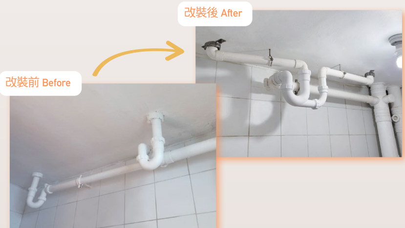
將為約1萬個現有單位安裝「W型」聚水器。 The drainage pipes in around 10,000 rental units will be fitted with W-trap system.
