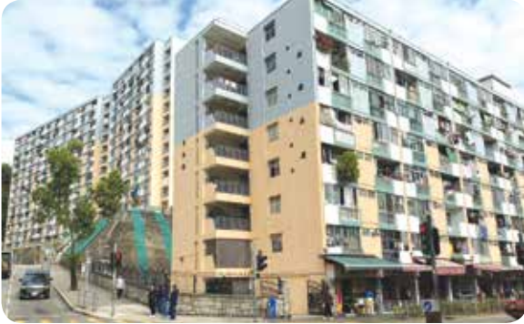
觀塘花園大廈二期的燕子樓及喜鵲樓的空置單位將用作「暫租住屋」，冀為緩和市民在輪候公屋期間的住屋需求。 Vacant apartments in Yin Chee Lau and Hay Cheuk Lau of Kwun Tong Garden Estate II will be converted into transitional housing units to address short-term public housing demands.
